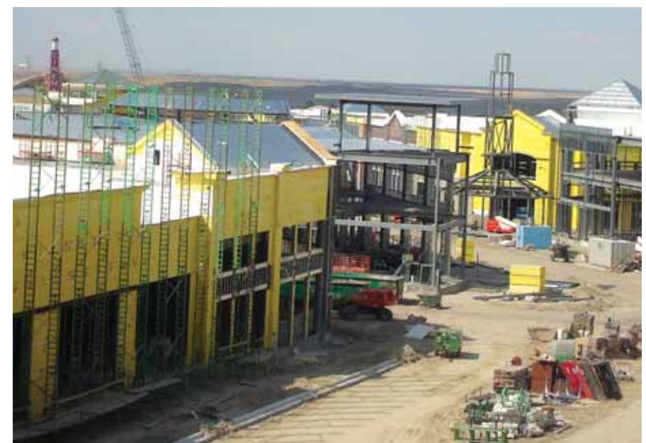
Main Street construction incorporates high-quality materials and a variety of exterior skins on the retail buildings, including masonry, metal panels, ceramic tiles and EIFS.
